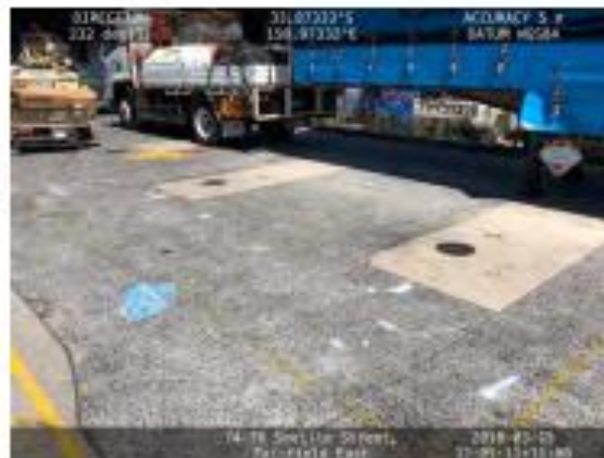
UST mark up utilising ground penetrating radar.
